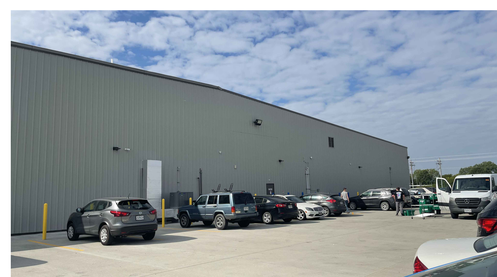
REFERENCE PHOTO - EXISTING BUILDING NORTH ELEVATION
