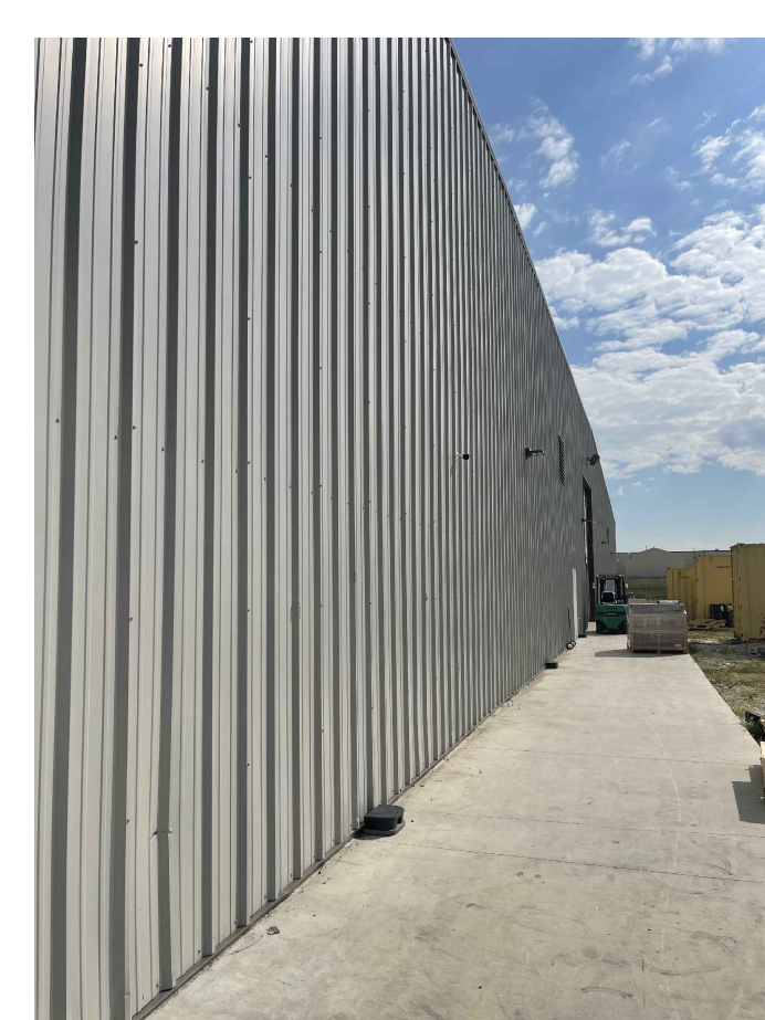
REFERENCE PHOTO - EXISTING BUILDING SOUTH ELEVATION
